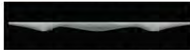
Figure 2.18: Concrete beam made with fabric formwork
